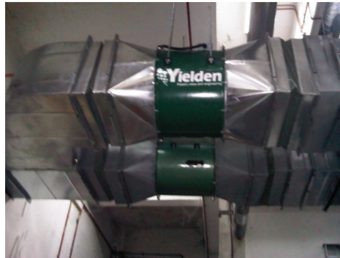
Ventilations fan and ducting works
